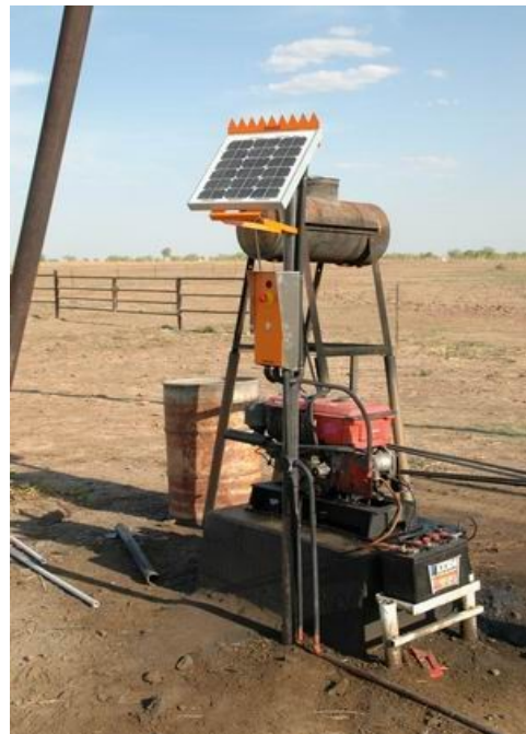
Outdoor pole mounted installation with supplementary power kit.
