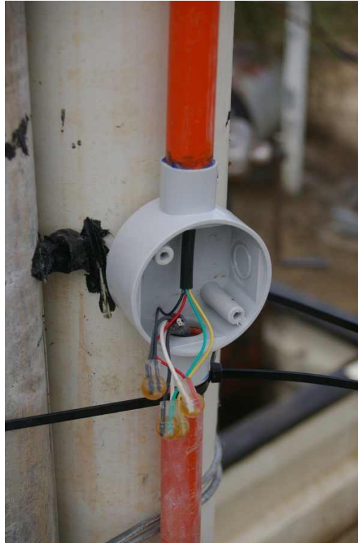
Multiple device type cable being spliced using the suggested connectors
